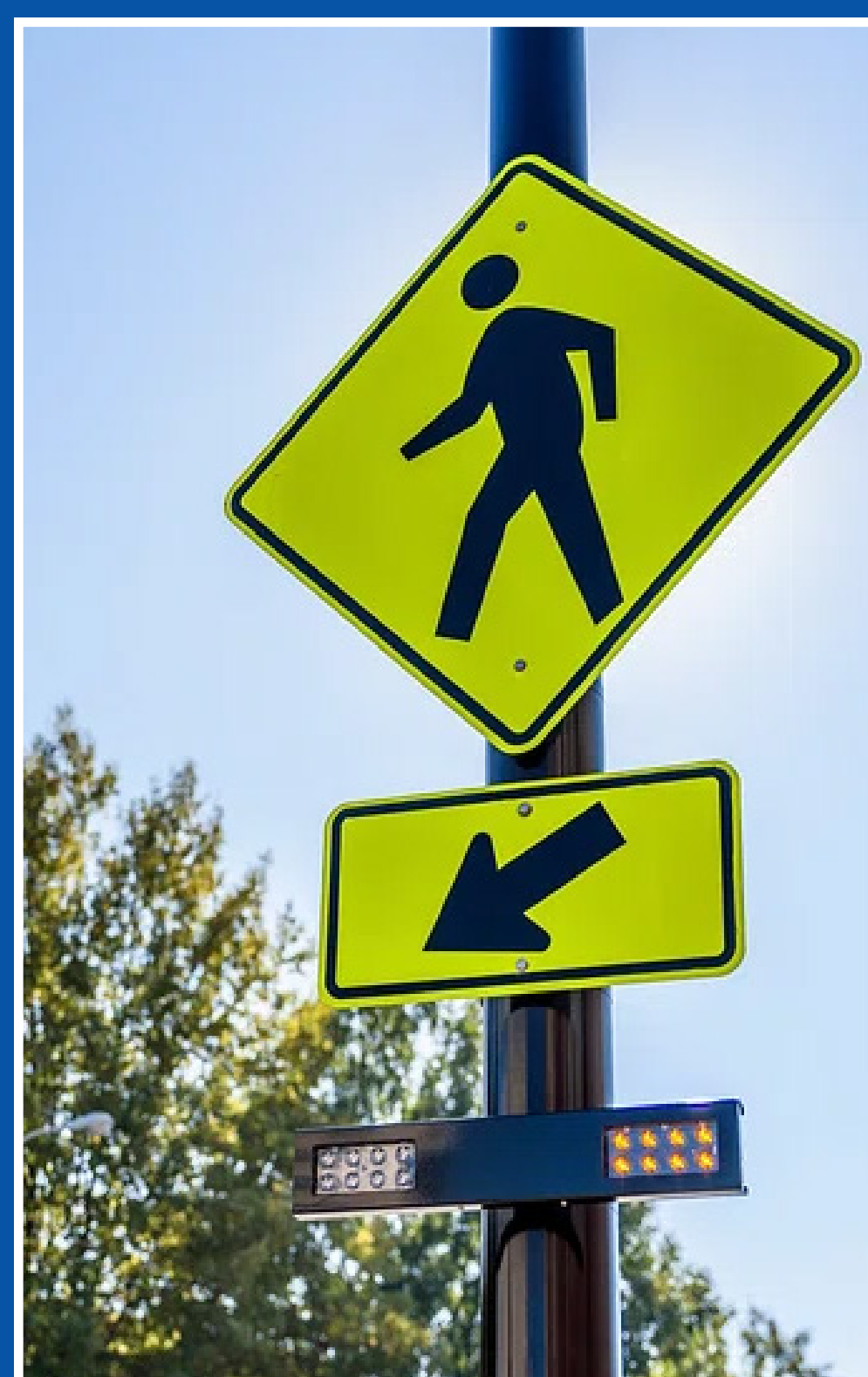
Rectangular Rapid-Flashing Beacons (RRFB)
